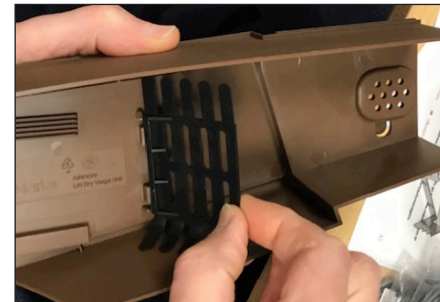
Fig. 5 – Position plastic filler piece at 45°
